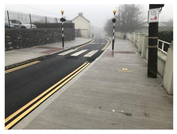
Figure 6.12: Raised Table Zebra Crossing Recently Installed on Cleamore Road
